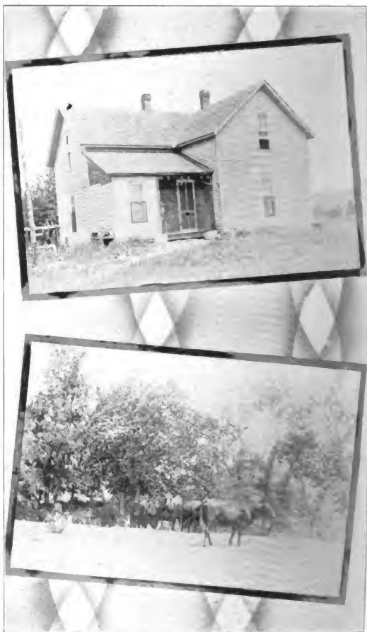
Residence and scene on Frank M. Darr's place, 2 miles east of Pure Air
